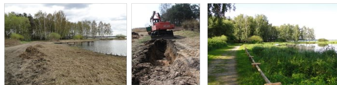
Denitrification walls + buffering zones (K. Izydorczyk)
